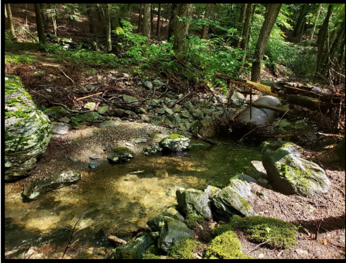
Figure 3. The plugged culvert on Burton Brook causes scouring of the streambank.
