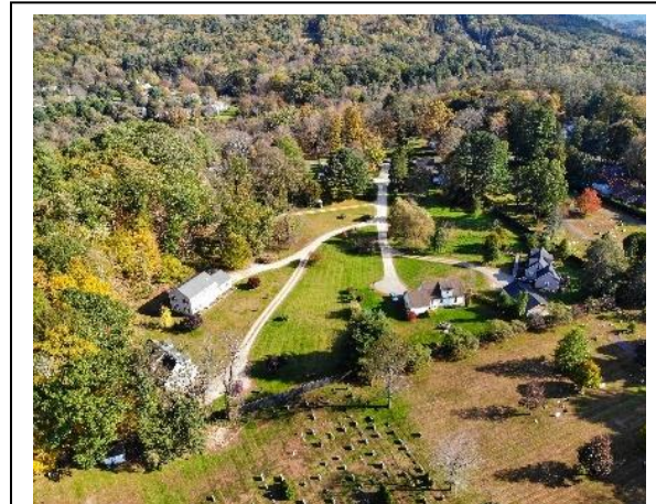
Dunham Drive – One of the first homeownership developments sponsored by the Salisbury Housing Trust Photo: Salisbury Housing Trust
