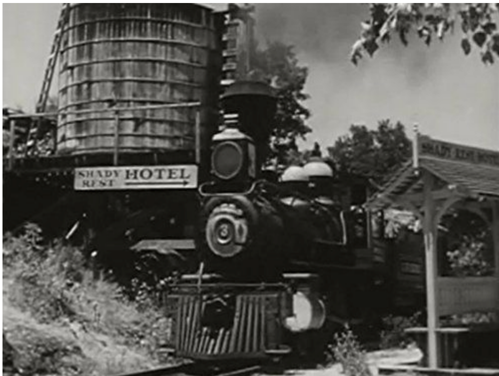
Figure 1 water tower more suited for swimming and trains
